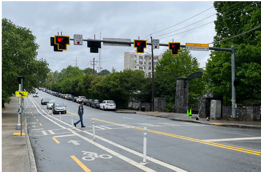
HAWK crossing of a road with cycletrack - 10th St NE (Atlanta, GA)
