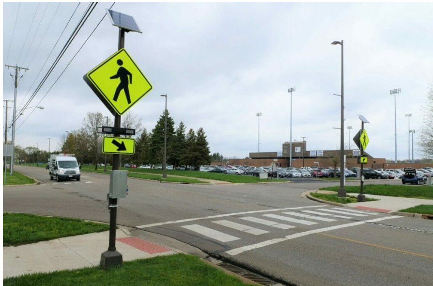
Rectangular Rapid Flashing Beacon crosswalk
