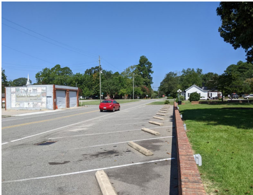
N Baker St – angled street parking, brick retaining wall
