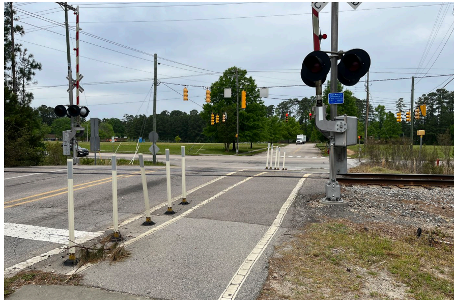
Railroad crossing within the existing roadway crossing and mast arm - Laura Duncan Rd (Cary, NC)
