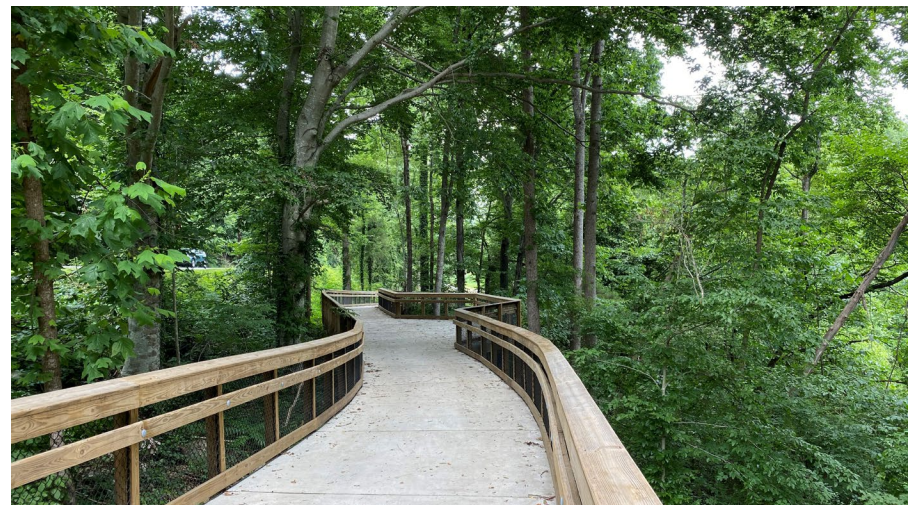
Concrete deck boardwalk - Toby Creek Greenway (Charlotte, NC)
